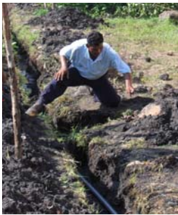
Laying the new waterlines
